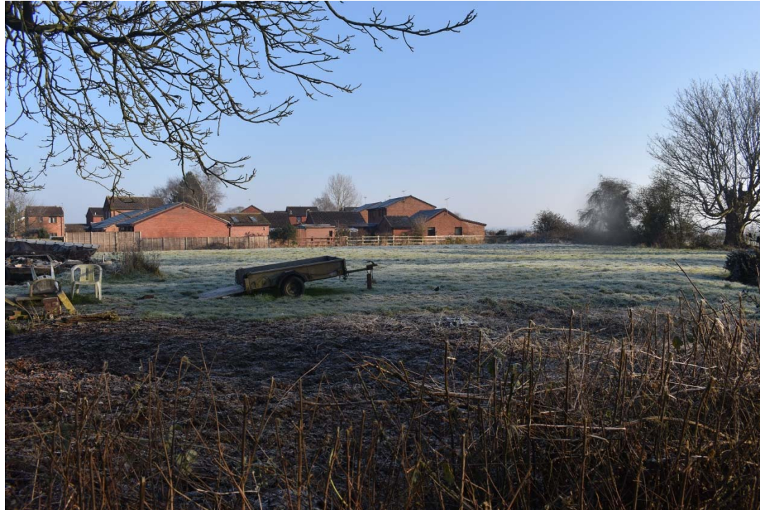
SCD003 - Site bounded on the north by single story houses
