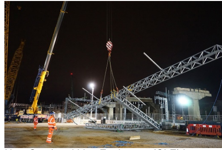
New Overhead Line Equipment (OLE) is installed
