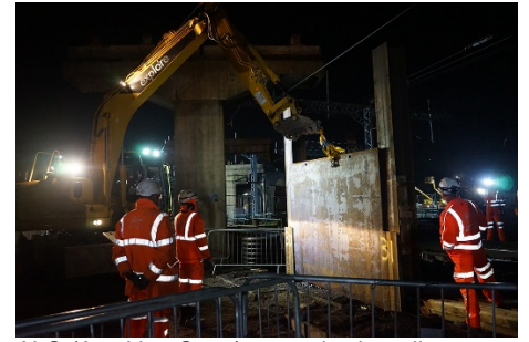
ALO (Any Line Open) protective hoarding is piled and installed
