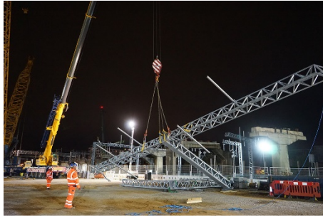
New Overhead Line Equipment (OLE) is installed
