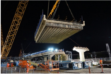
A span is lifted from Bletchley Flyover
